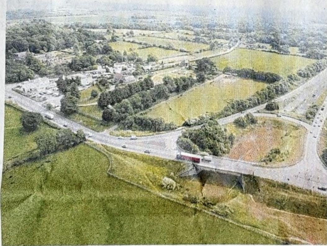
The Crossbush junction along the A27
